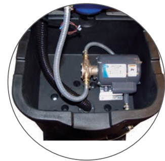
Discharge pump located in equipment bay rather than recovery tank
