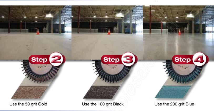
Use the coarse 50 grit Gold polymer and proceed as you would with your regular floor cleaning routine. After a few passes using the 50 grit, the system progresses to the next grit.
